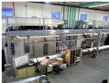
Building energy management systems
